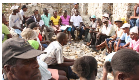
In Veyon, Haiti, Organizasyon Kominotè Fanm Veyon [Women's Community Organization of Veyon] (OKFV) community members meet on the construction site of a new produce storage facility they are building with IAF support.
